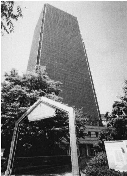
Fig. 4. Umeda Center Building (37 000 h operation).
